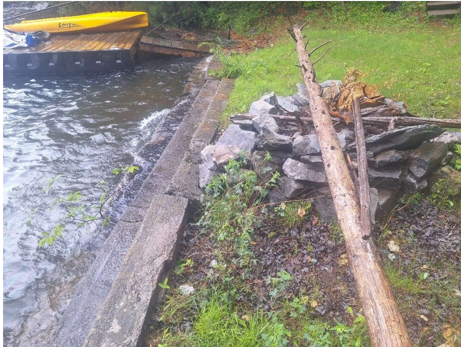
Photo 2: Lawn community and fire pit on the Site, bordered by concrete steps along the shoreline.
