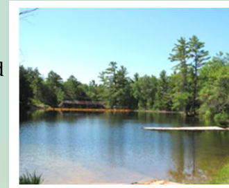
Mississagua Lake Dam
