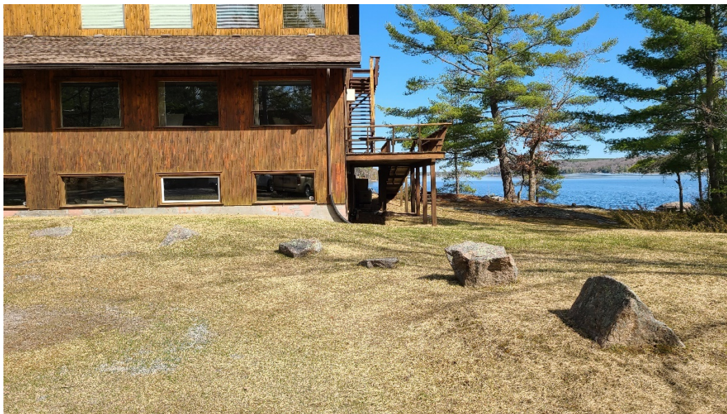
Photo 2 – Looking east from the detached dwelling to the southwest corner of the Gallery building
