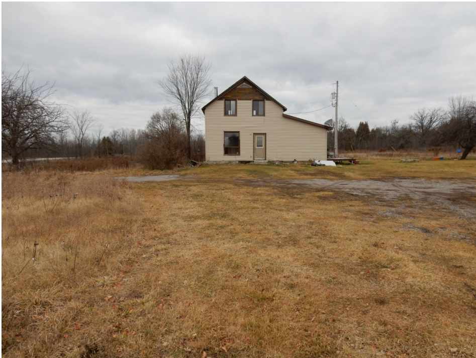
Image 1: View N towards recently abandoned house showing gravel driveways.
