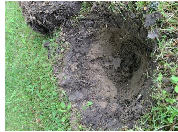
IMAGE 3 COMPLETED TEST PIT
