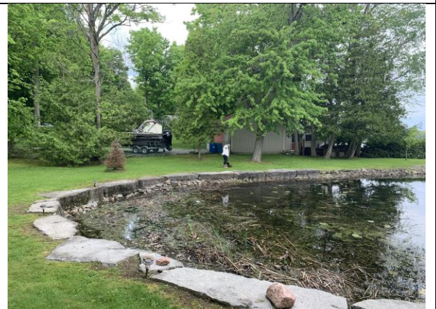
IMAGE 6 CREW CONDUCTING TEST PITTING AT 5M INTERVALS AND BUCKHORN LAKE
