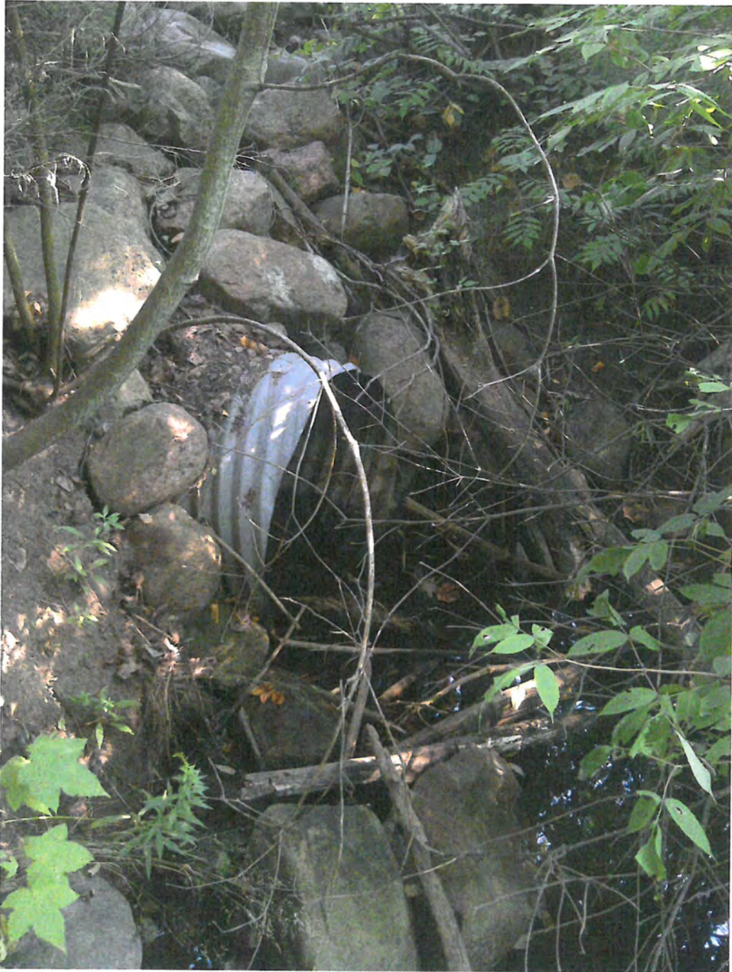
Adam & Eve Road Culvert – Outfall
