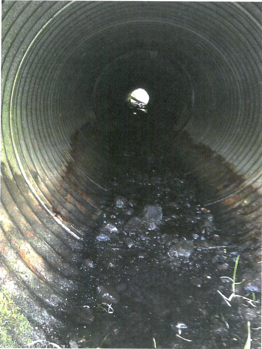
Adam & Eve Road Culvert –view from upstream to downstream
