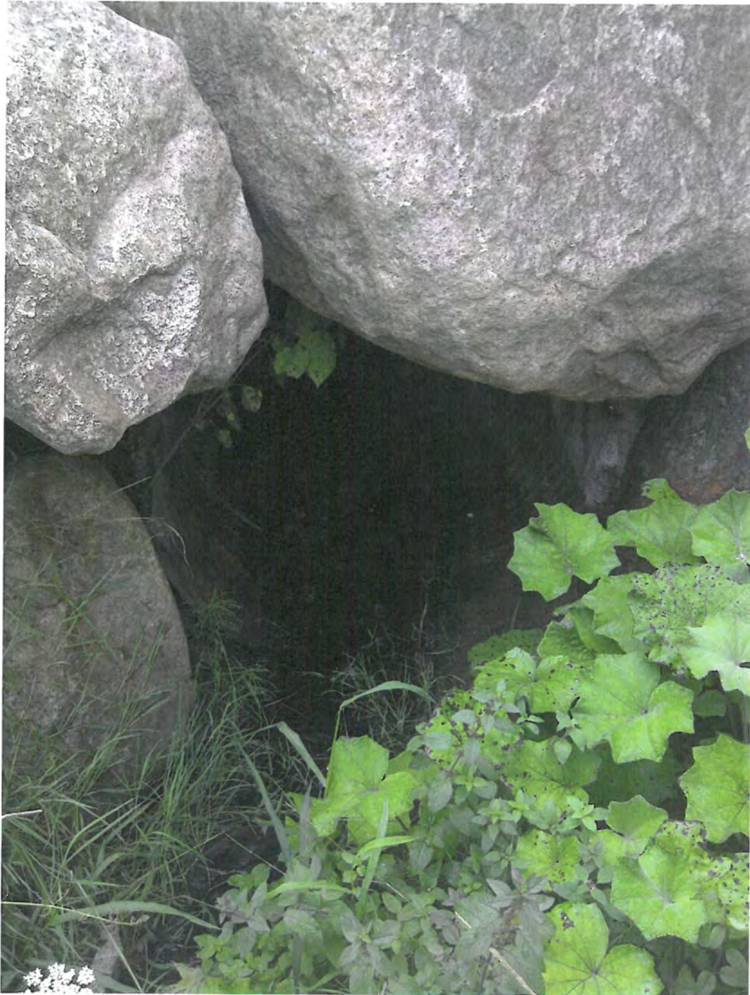
Adam & Eve Road Culvert – North inlet
